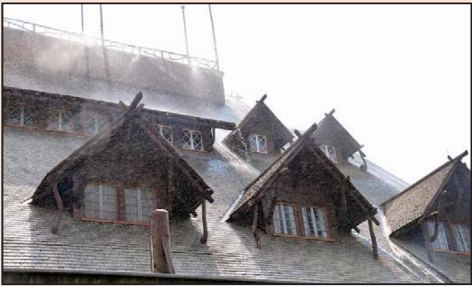
Old Faithful Inn, Yellowstone; testing the rooftop system in 2020 as fire was burning not far away.
