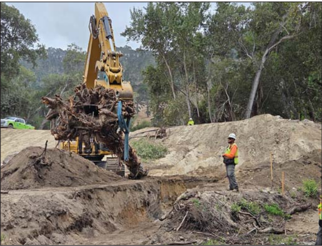
Workers using heavy equipment on a habitat restoration project along Carmel River need to pay close attention to the wildlife.
