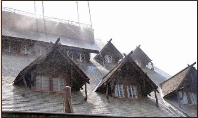
Old Faithful Inn, Yellowstone; testing their rooftop sprinkler system over the wood shake roof in 2020 as fire was burning not far away.
