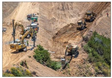
Work continues to reopen Highway 1 at Regent Slide in Big Sur, where 2,000 steel rods were recently installed to stabilize the site.
