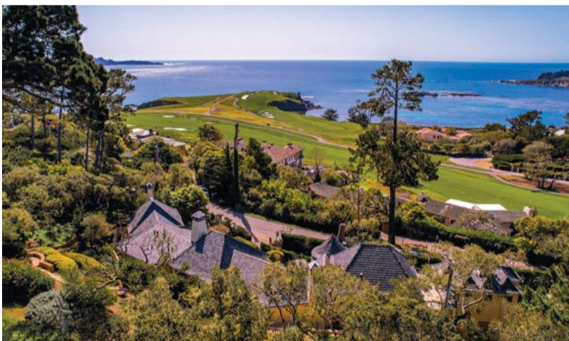
Ocean, Stillwater Cove & Golf Course Views from Every Room
