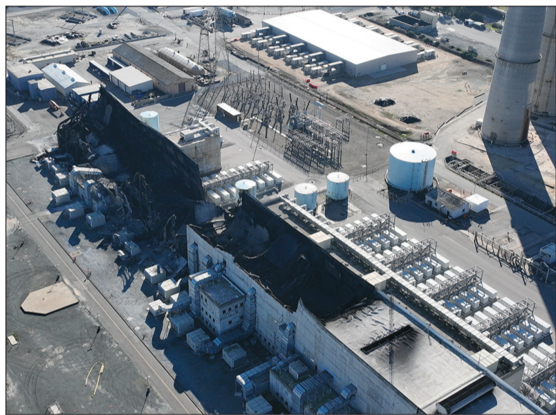
A blackened hole (above) is all that’s left of a Vistra Energy facility in Moss Landing after Thursday’s disastrous fire, which forced evacuations, closed Highway 1 and lit up the sky for miles around (right).
