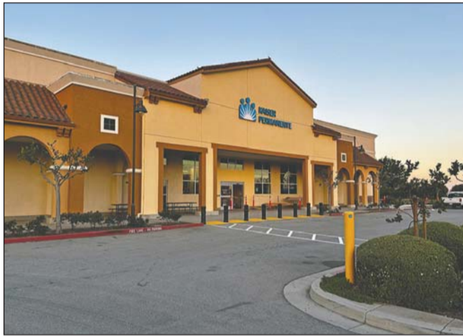
This new building, which formerly housed a Babies "R" Us retail store, is being converted into a new medical facility for Kaiser Permanente. The clinic is set to open Jan. 2, 2025.
