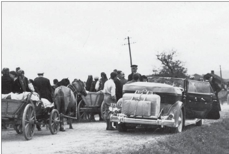
PHOTOS/COURTESY LAVINE RESTORATIONS
