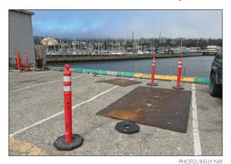
Steel plates like this one have been placed to cover dangerous holes in the decking on Monterey's Wharf No. 2
