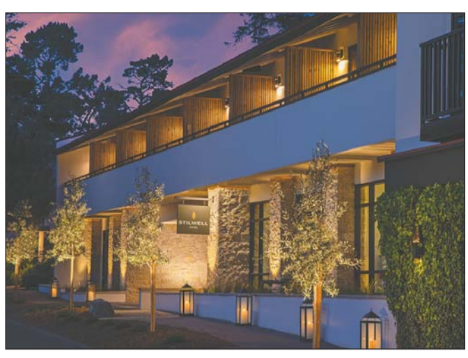
After a long time looking drab, followed by more than two years of construction, the remodeled and rebranded Stilwell Hotel quietly opened this week.
