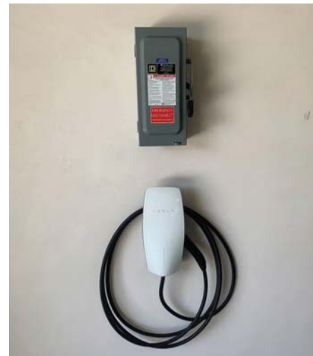
Charger installation for electric vehicles is among Craft's specialties.
