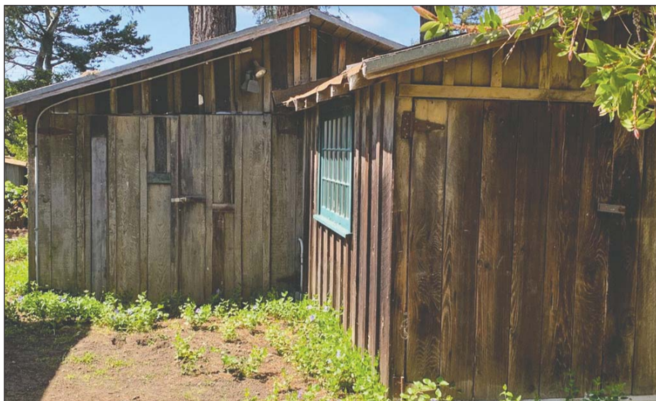
Built nearly a century ago, a former garage at the Cherry Center for the Arts is getting new life as an art studio.
