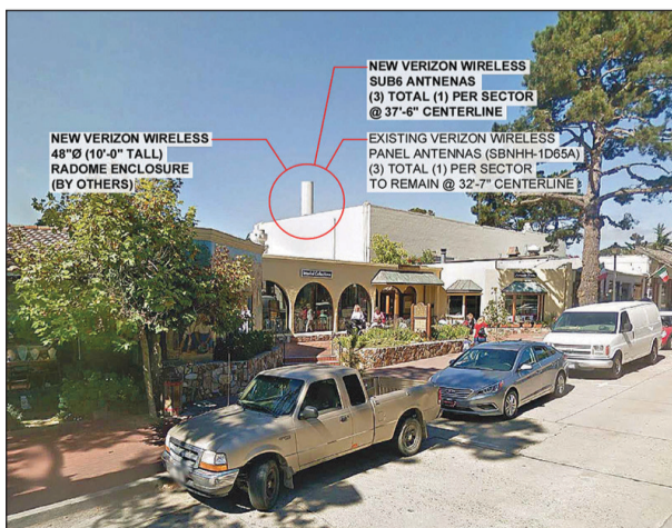
A graphic provided by Verizon shows a wider, taller fake smokestack on the roof of the Doud Arcade.
