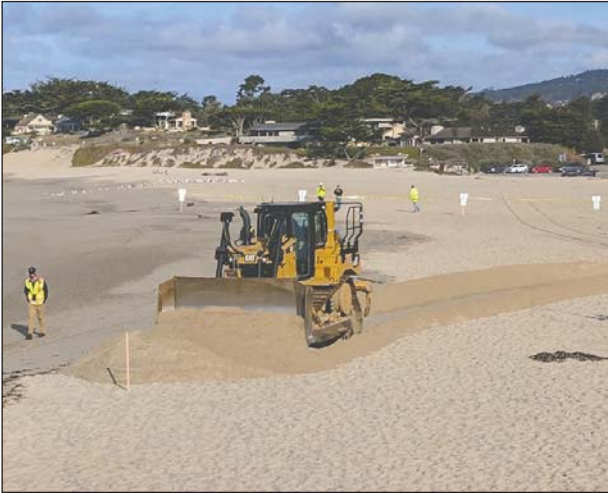
In 2019, a county worker (left) uses a bulldozer to cut a channel in the Carmel River Lagoon Sandbar to release water that was threatening homes. Early this year, county workers (right) respond to flooded streets and homes near the lagoon.
