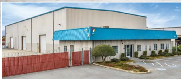
1650 Lana Way, Hollister -Main Warehouse is 15,100 sq ft
