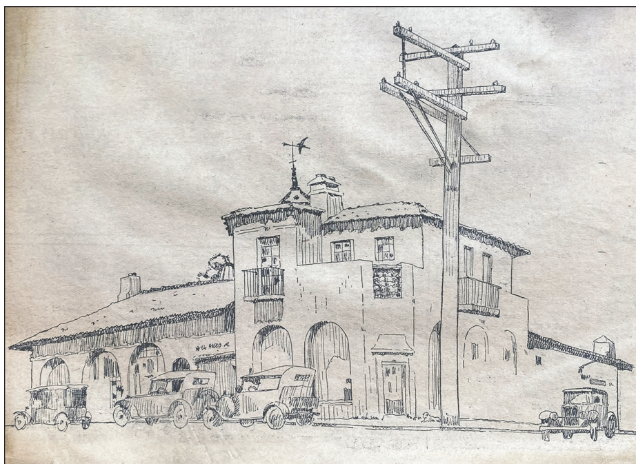
This drawing of the El Paseo building at Dolores and Seventh first appeared in the April 27, 1928, Carmel Pine Cone. Lewis Merrell had the telephone pole removed and the lines undergrounded in 1929. Today, the building is owned by Rod Dewar and Jean Mouton and houses the Little Napoli restaurant.
