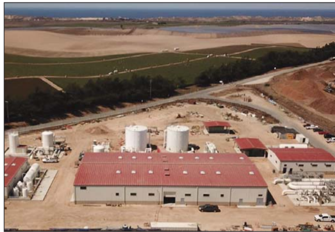
The Monterey One Water facility near the Marina landfill is the home of an advanced water purification facility that will transform wastewater into drinking water for Monterey Peninsula residents.
