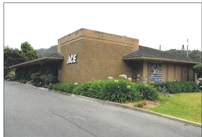
PHOTO/WALD, RUHNKE & DOST ARCHITECTS
