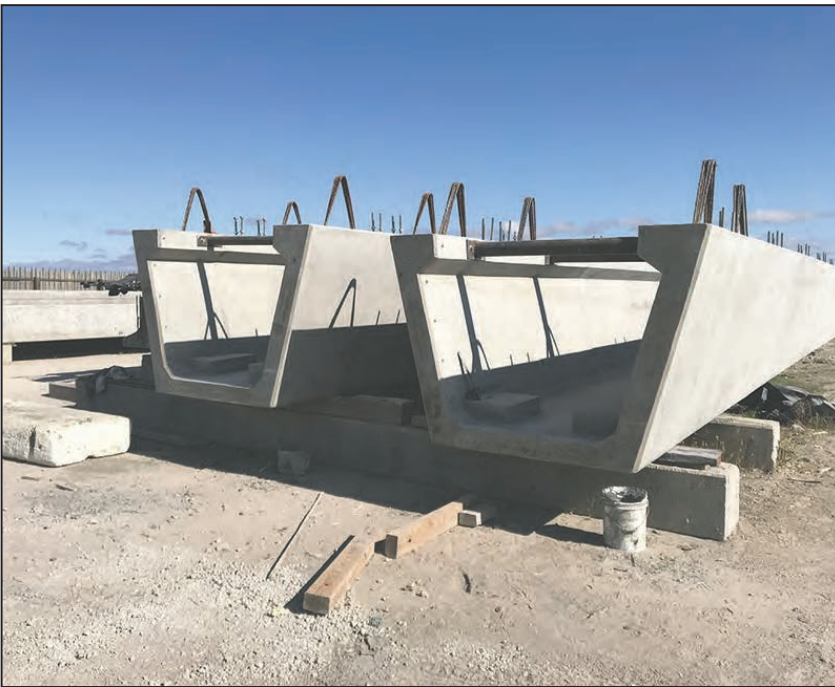
Two precast concrete girders – each one resembling a giant trough – will be installed over Highway 68 near the Monterey Fairgrounds next week. (Caltrans photo)
