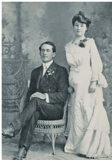
1904 M.J. Murphy and his wife Edna settled in Carmel. He built a one-room home which still stands today on 9th & Monte Verde. M.J. started as a carpenter but expanded his business to cover all aspects of his trade.
